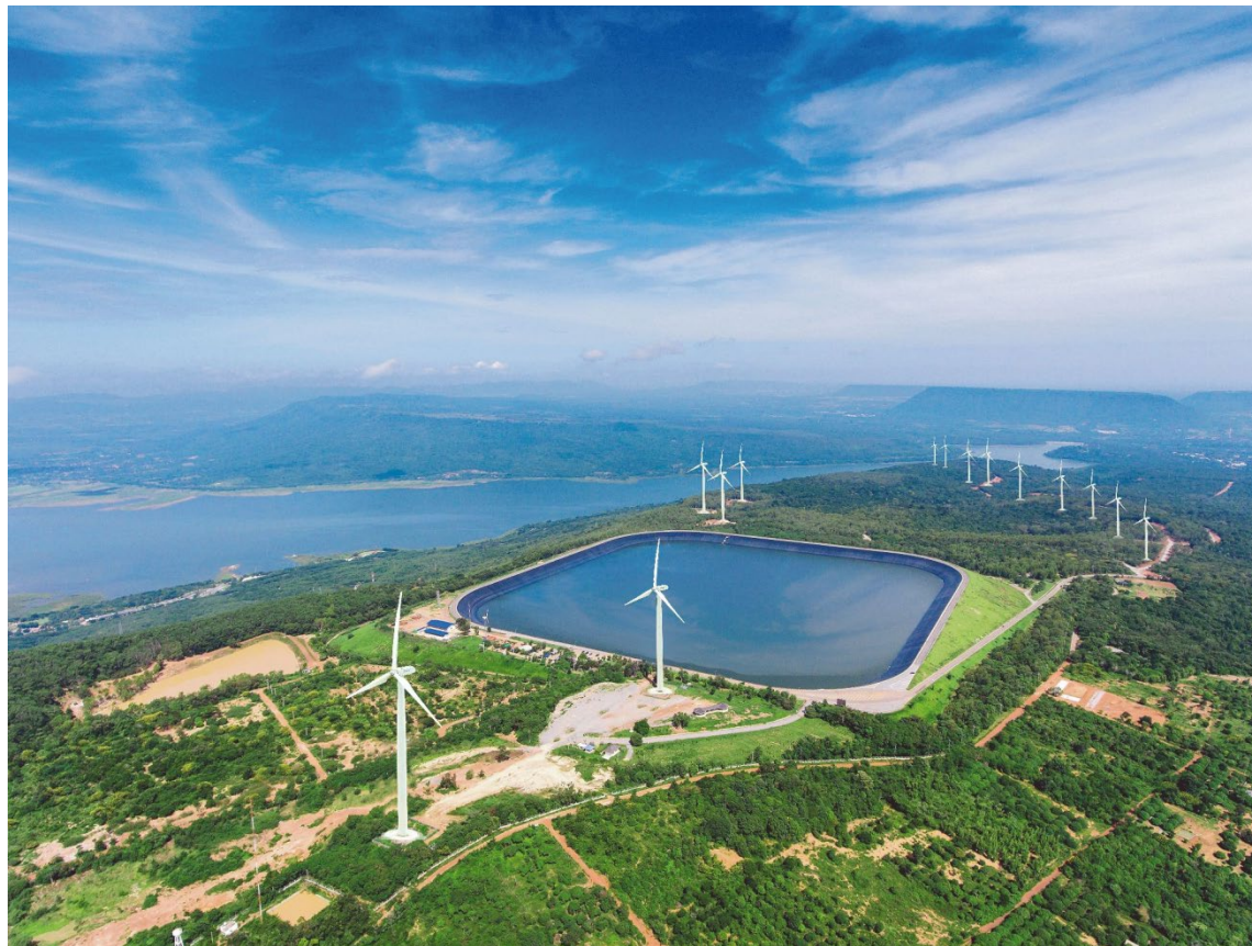
1000-MW Lamtakong Jolabha Vadhana Power Plant, Nakhon Ratchasima, Thailand
