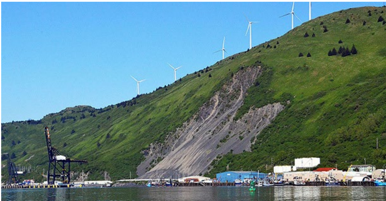
2-MW FES system at Kodiak Island, Alaska, USA
