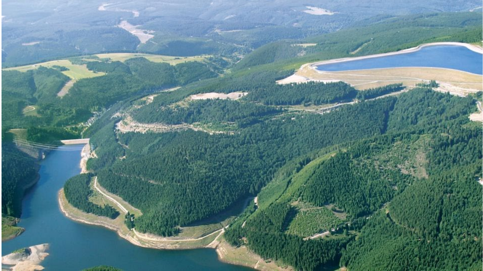
1060-MW Goldisthal PHE plant, Goldisthal, Germany
