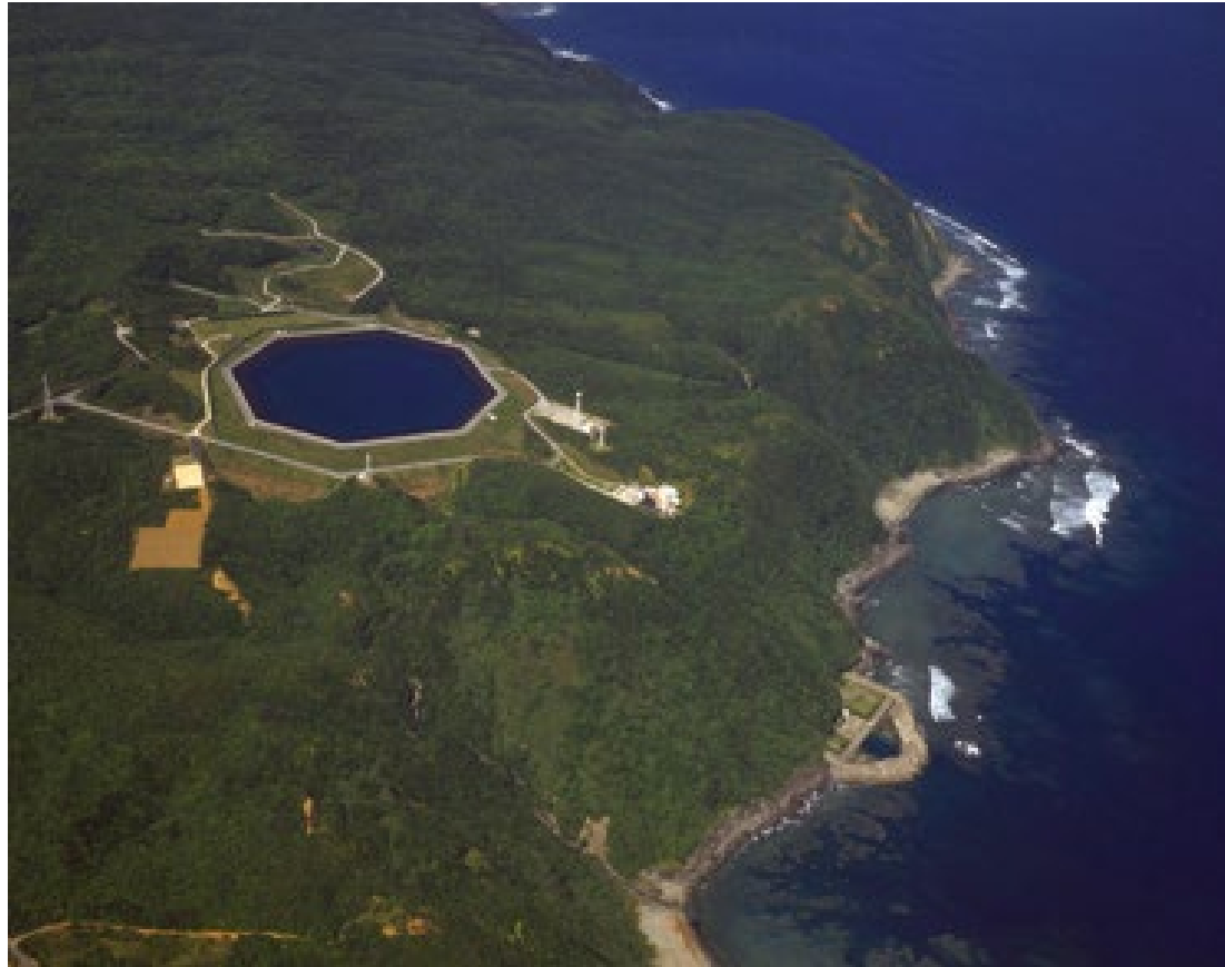
30-MW Okinawa Yanbaru Seawater PHES plant, Okinawa, Japan
